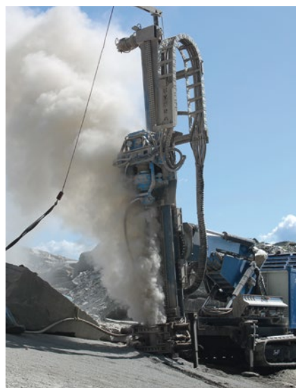
VD100 drilling in medium-hard rock, 100 m deep, hole diameter 135 mm, flushing with air
